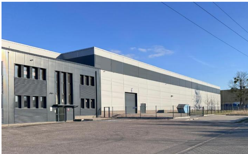
Figure 4. Example of homogeneous sandwich panel used for industrial construction.
