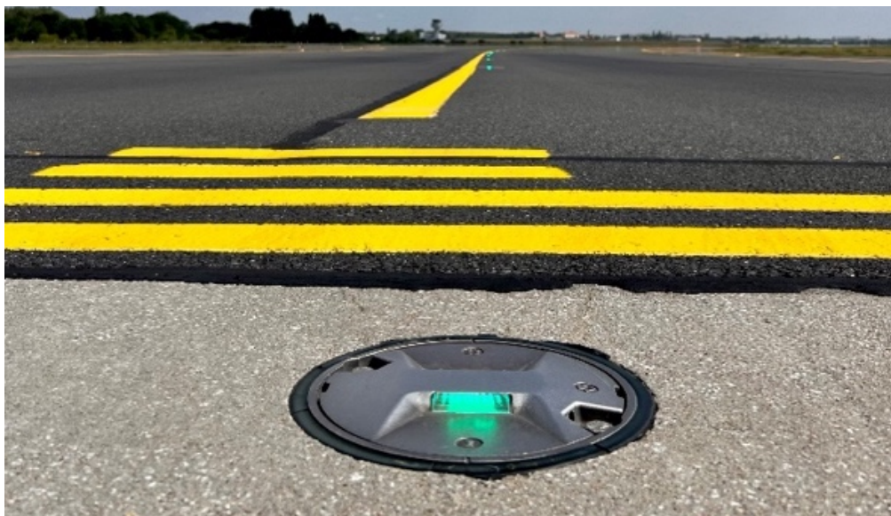
Figure 2-6 Airport taxiway centreline in-pavement lamp [41]
