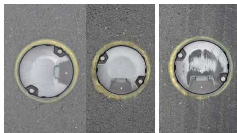
Figure 5-6 Examples of Touchdown zone lamp IDM4671 [40]
