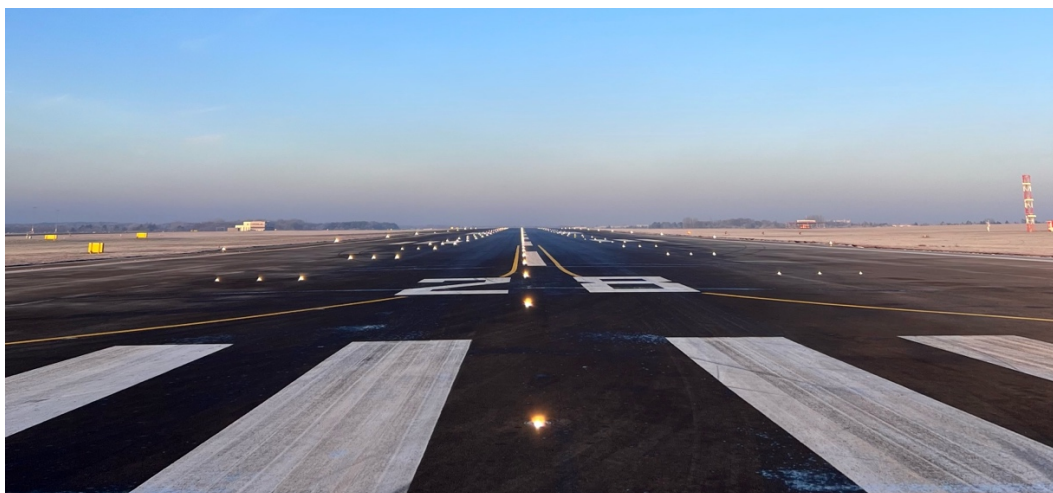
Figure 1-1 View at runway 28 at the Poznań–Ławica Airport with visible airfield ground lightning (AGL)
