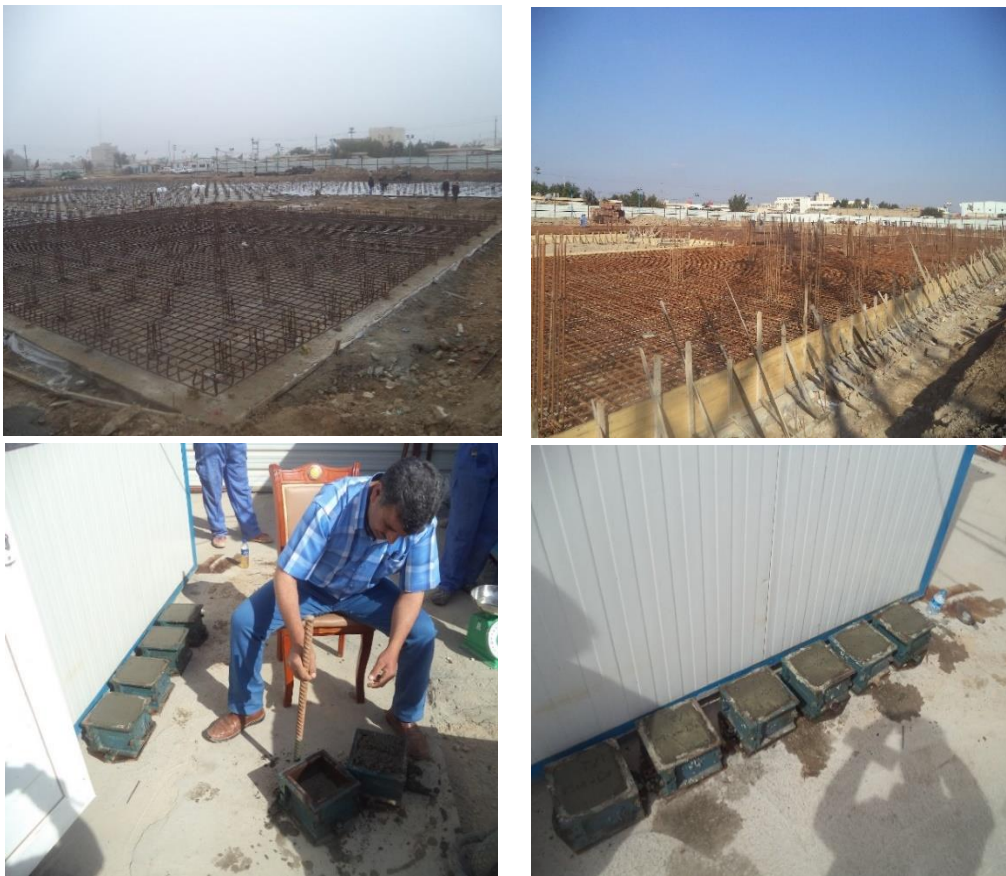
Figure 6.14 RMC compressive strength samples for foundations (six cubes) at 28 days [Researcher].
