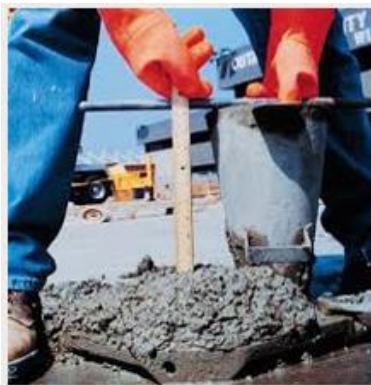
Figure 1.5 Accelerated Slump Loss (Slump test failure) [22].
