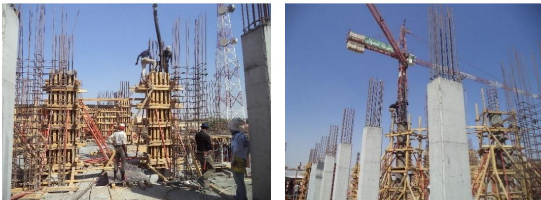
Figure 7.16 RMC compressive strength f_c (MPa) test samples for the building columns of the second floor, six test samples at age 28 days [Researcher].
