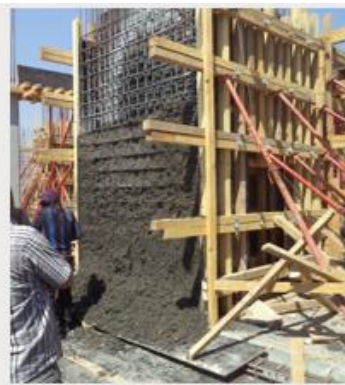
Figure 1.6 Faster Set Times Consistency & Air content failure [Researcher].
