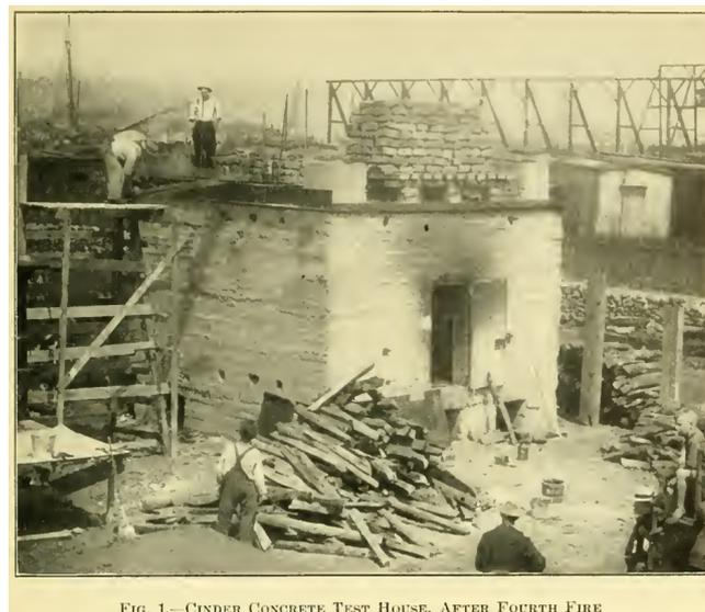
FIG. 1.— CINDER CONCRETE TEST HOUSE. AFTER FOURTH FIRE
